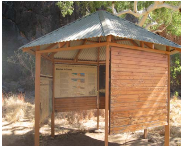
Interpretation Booth at Tunnel Creek.
